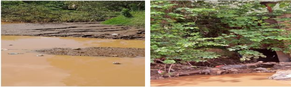
Figure 5: Siltation and erosion at upstream of the intake.
