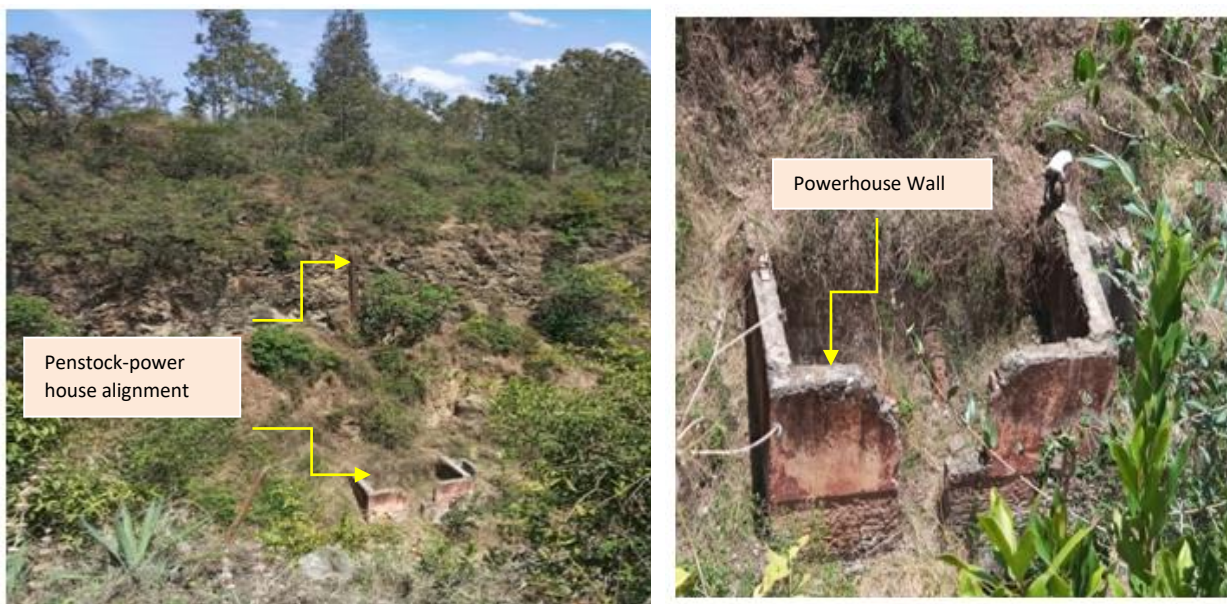
Figure 3: Showing Existing Penstock-Power House Alignment
