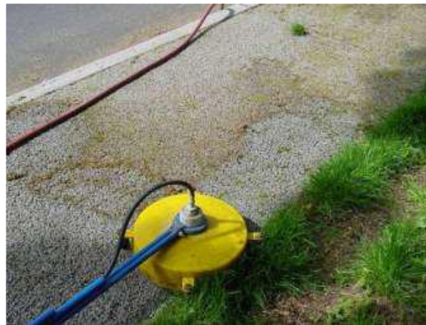
Fig. 5 - Vacuuming of pervious concrete pavement.
