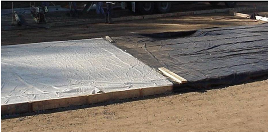
Fig. 4 - Curing of pervious concrete by plastic sheet covering.
