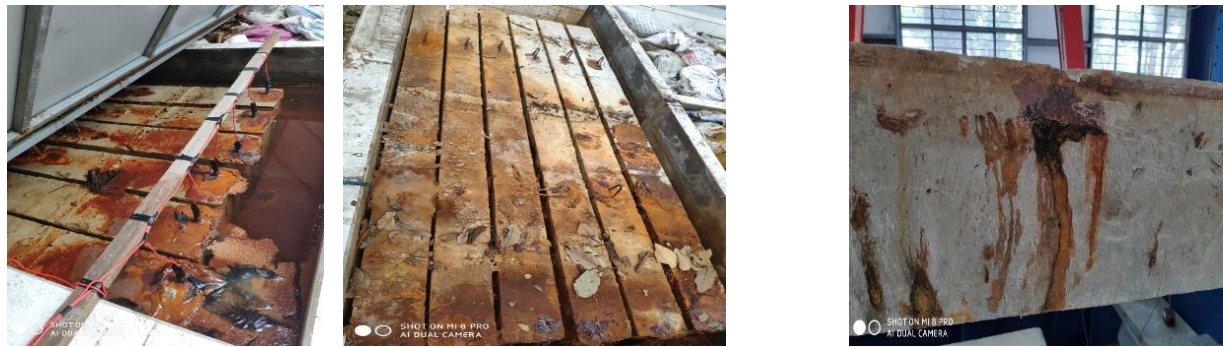
(a) Corrosion specimens
