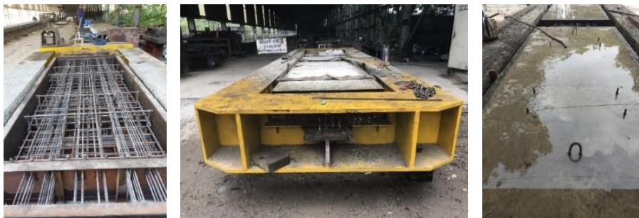
Fig. 4 – Production of PSCS sample in the factory
