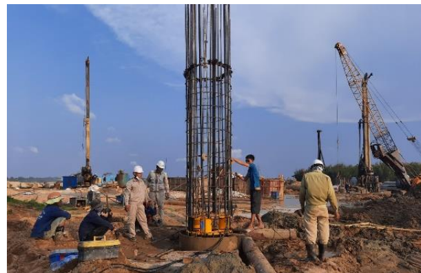
a. Test piles installation
